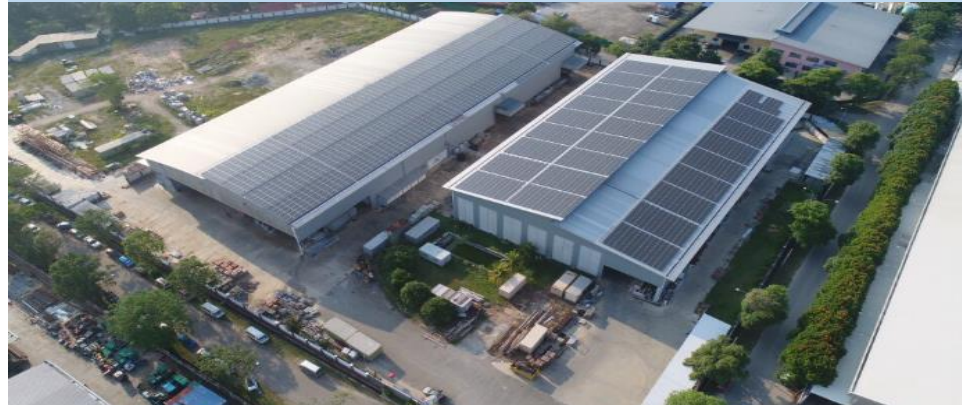
EPCC of solar PV system on factory rooftop under FiT programme
