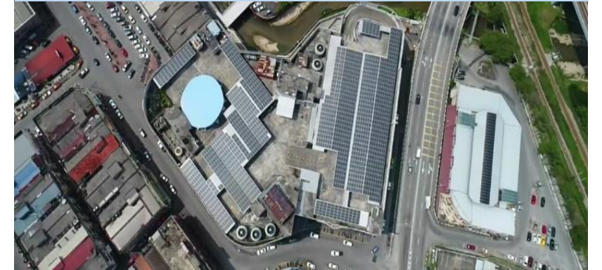
EPCC of solar PV system on shopping mall rooftop for the mall's self consumption in Kajang, Selangor
